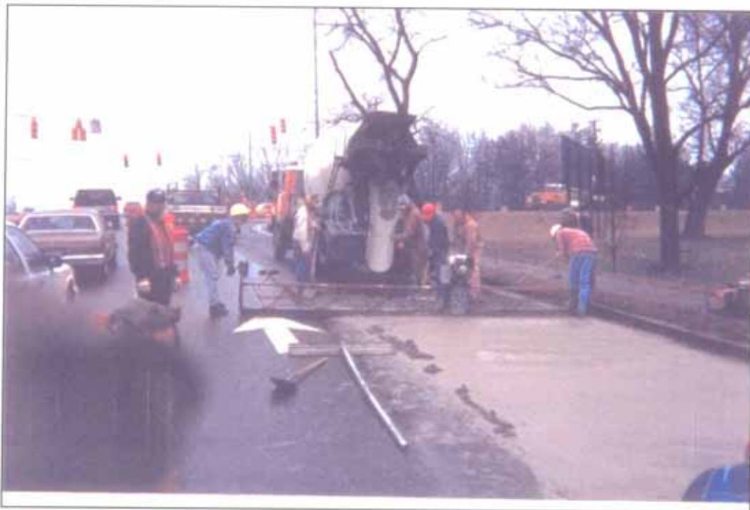
Wednesday morning - 1/12/94 Conventional methods were used to place the concrete
