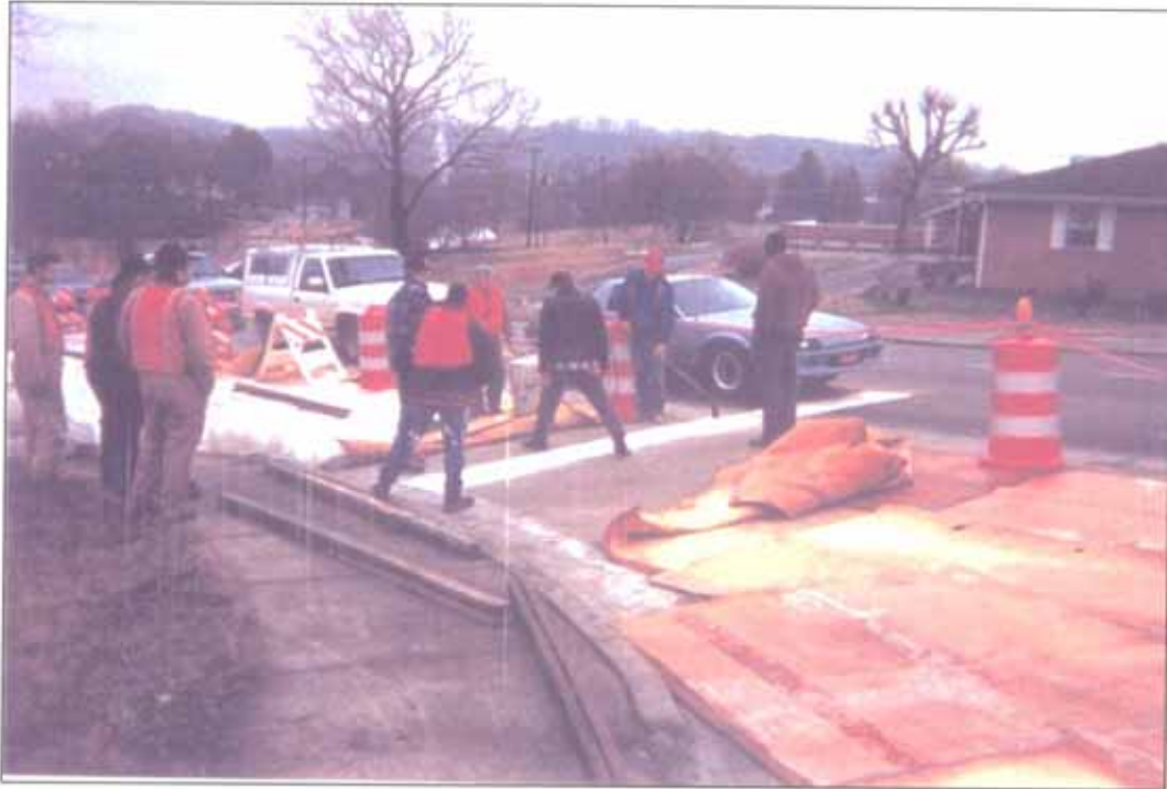
The inlay was covered with curing blankets overnight
