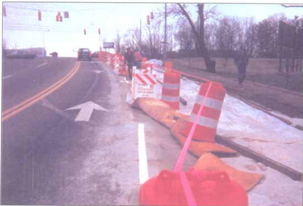
Lines were painted the same day the concrete was placed
